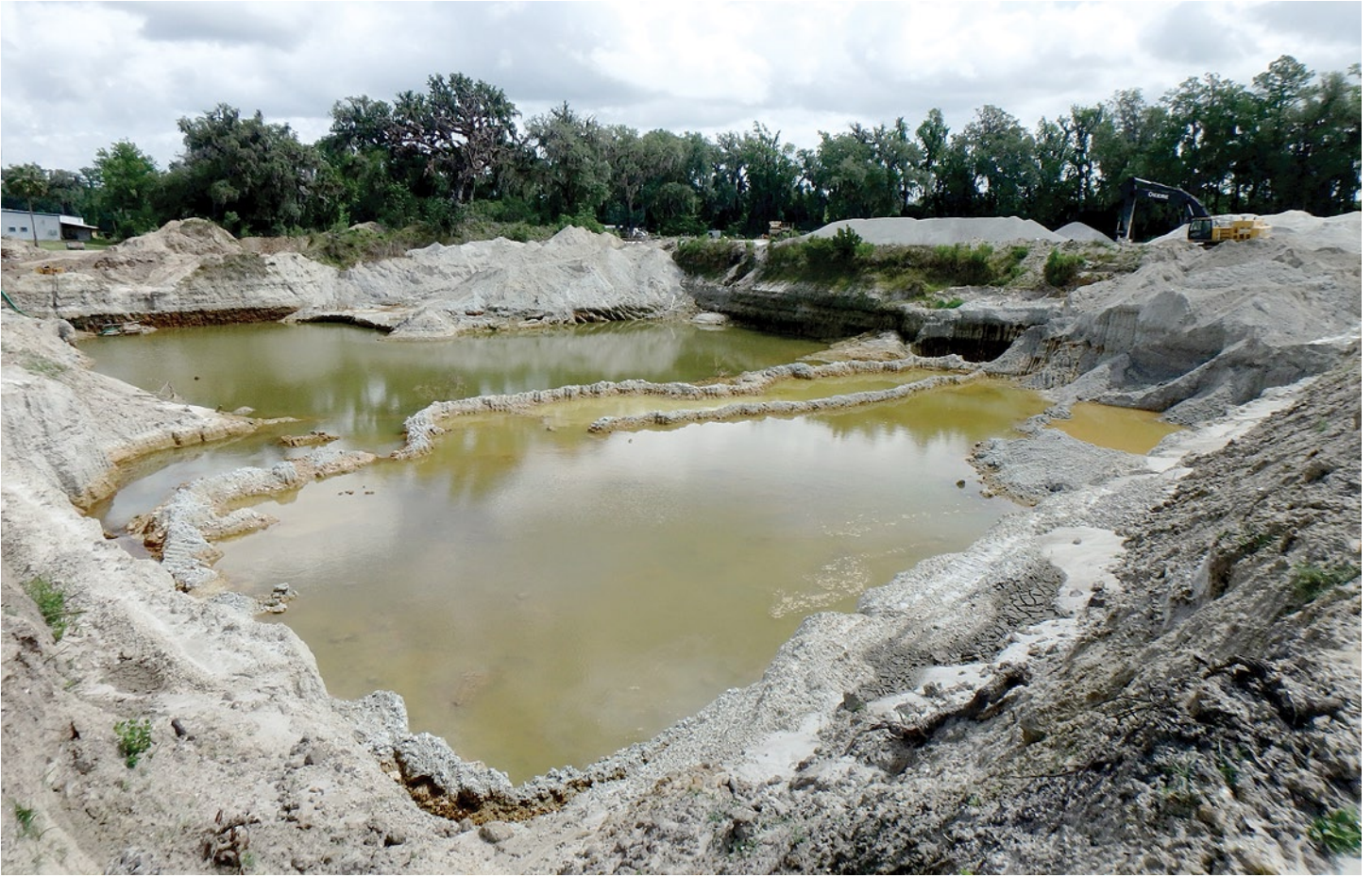
Figure 4. View of the recently de-watered Big Horse Aggregates Pit.
